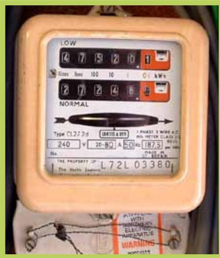
The top row keeps count of how much “off-peak” energy you have used, take away the previous “LOW” reading from the new “LOW” reading.
